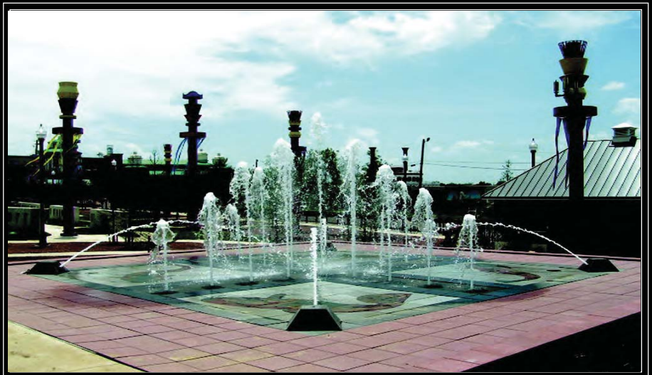
# 27 - 3 PEM 953's PEM E40 Catfish Fountain Vicksburg, Mississippi USA
