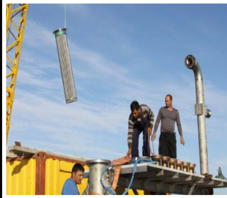
PEM 12"Flow Straightener Installion
