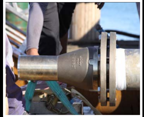
PEM 876 C being installed
